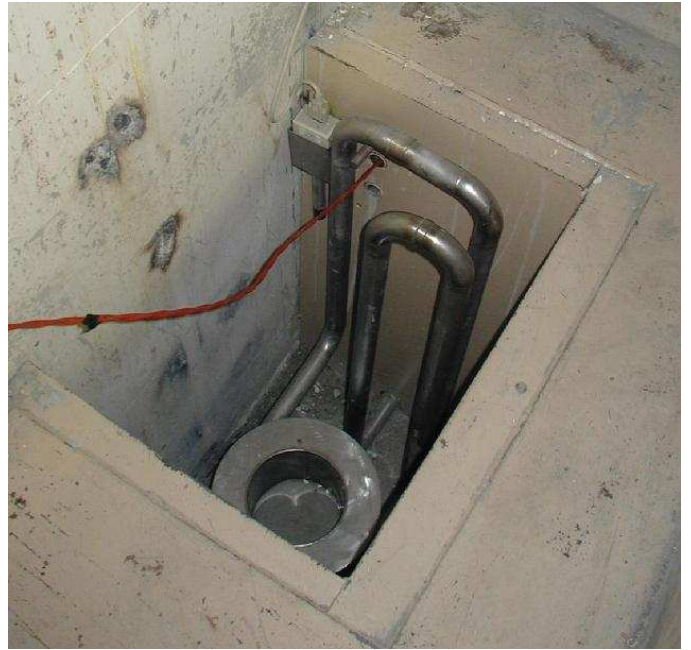
Fig. 4. A look into the radiation shielding bunker. The round structure inside is the bath designed to hold the neutron generator.
