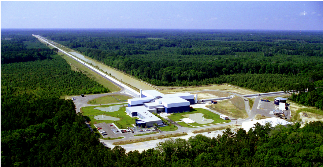
Figure 1.6: Aerial view of the LIGO observatory in Livingston, Louisiana (USA). The large corner building hosts the laser generator and one of the main mirrors of each arm. The beam pipes extend for 4 km in each direction covered by the arched, concrete enclosures seen in this picture (Credit: LIGO Laboratory).
